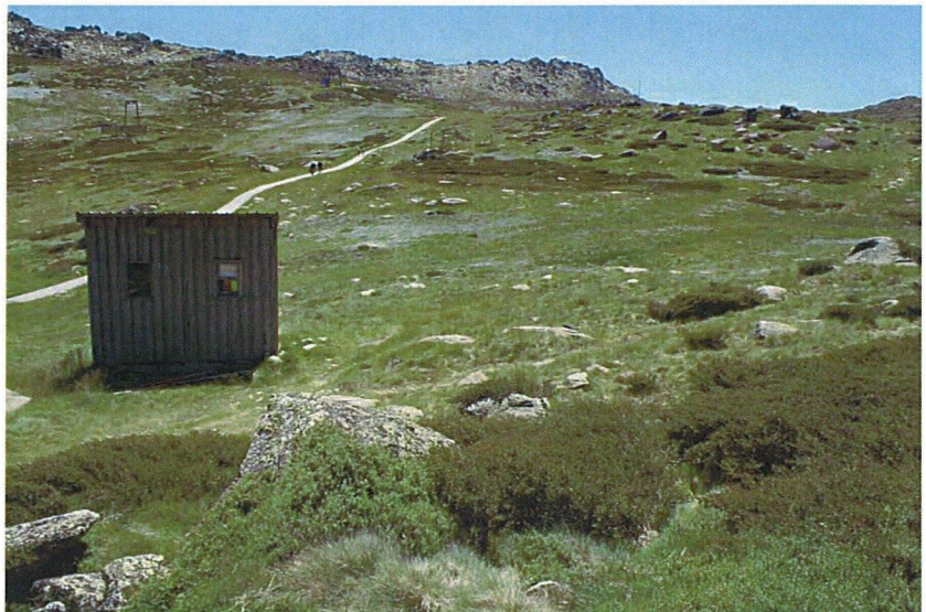
Figure 2: Location of the proposed communications hut – view towards the west
